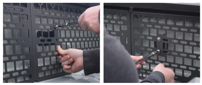
9. Using ¼-20 x ½" screws and washers attach panel to lower bracket. Leave screws loose.
